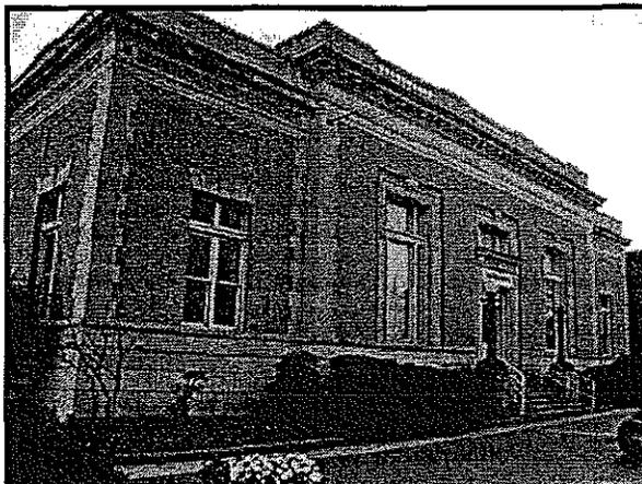
*The (former) U.S. Post Office on Hay Street is built on a stone foundation. The brick walls are accented by stone quoins and cornices.*
