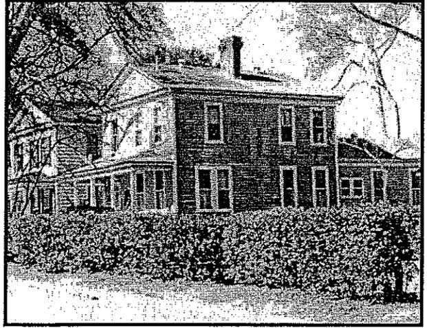
*The addition behind this historic structure is appropriately located on a secondary facade and of smaller scale than the principal building.*
